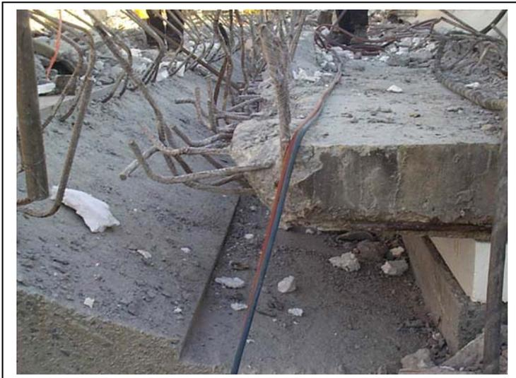
*Broken out edge of old Loftus St Bridge with underslung cantilever from new bridge, Perth.*
